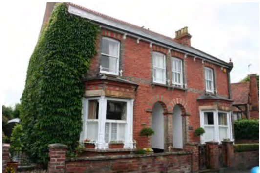
Grasmere and Moorlands 2-storey semi-detached villas with barley-sugar columns supporting bay cornices, metal railings on sills, ornate brackets supporting roof.
