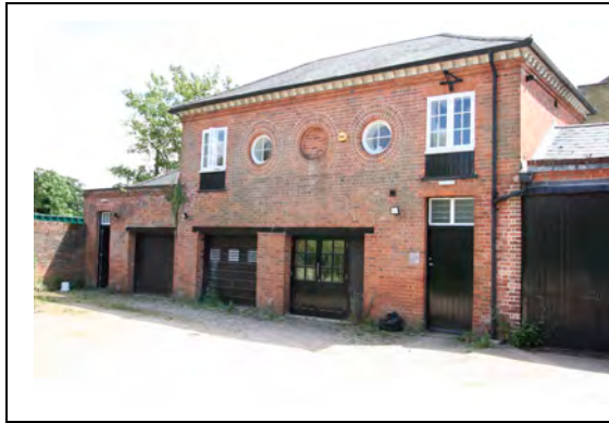
The Grove coach-house Late 18 th - or early 19 th -century, brick-built coach house with associated stabling for The Grove.
