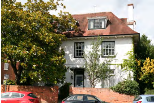
Moor Cottage 1830 3-bay house enlarged and modified in arts and crafts style at turn of 20 th century.
